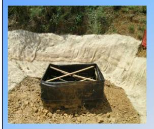
The same inlet after protected with a silt fence and frame for structural support.
